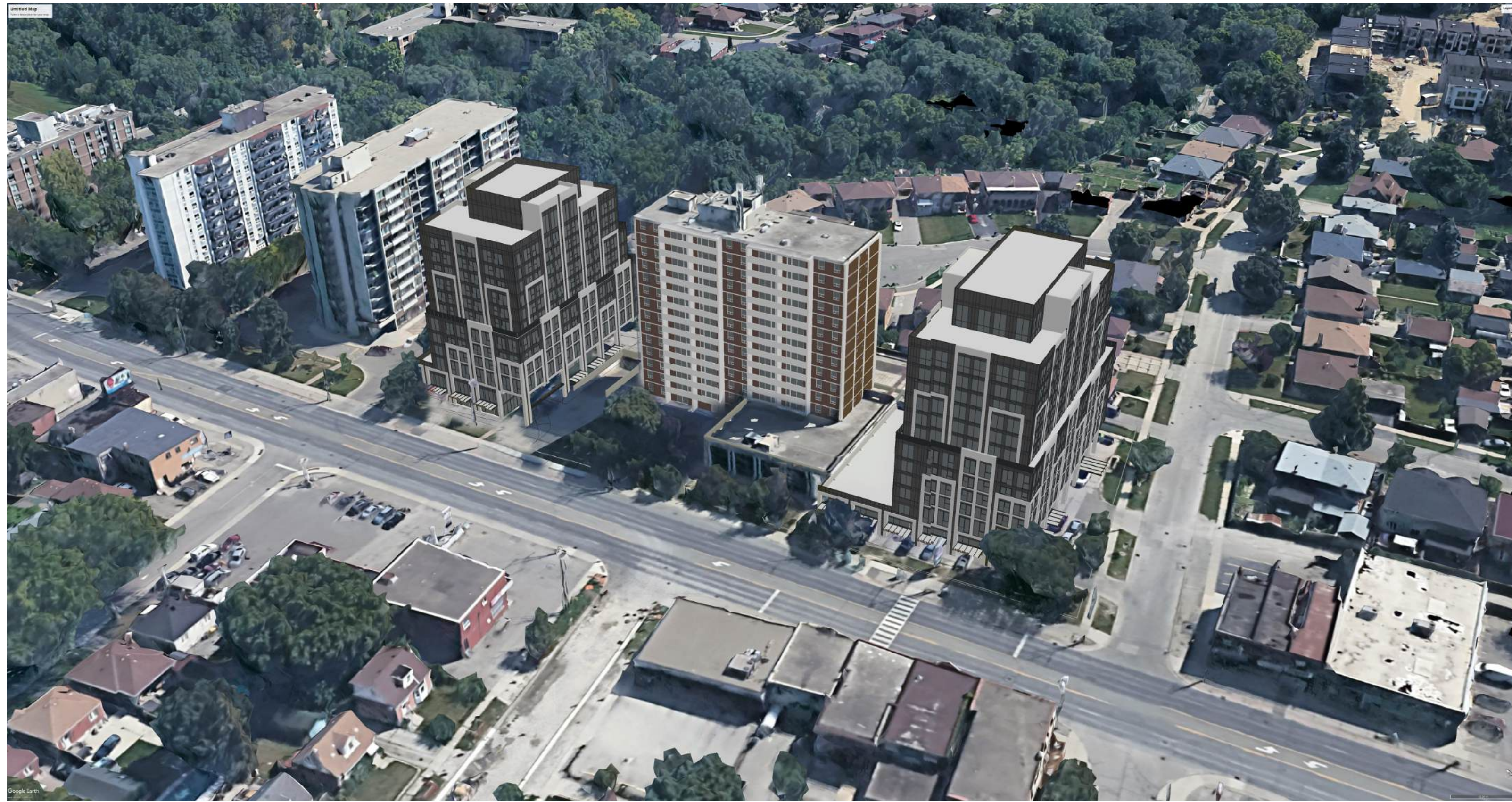
AERIAL VIEW FROM SOUTHWEST TO NORTHEAST
