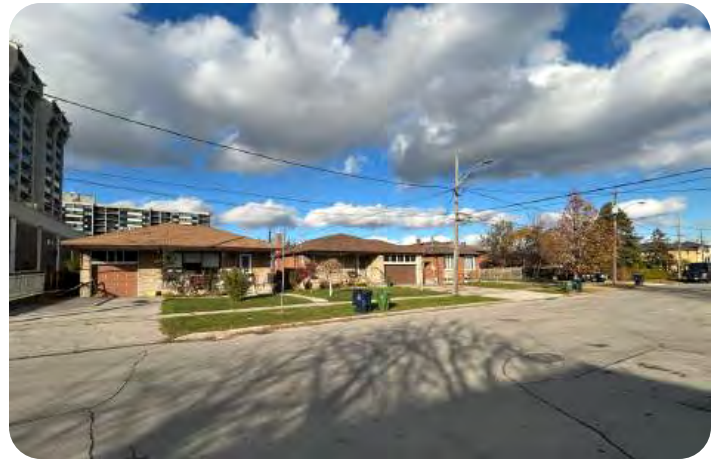
16 to 20 Marshlynn Avenue, looking northeast
