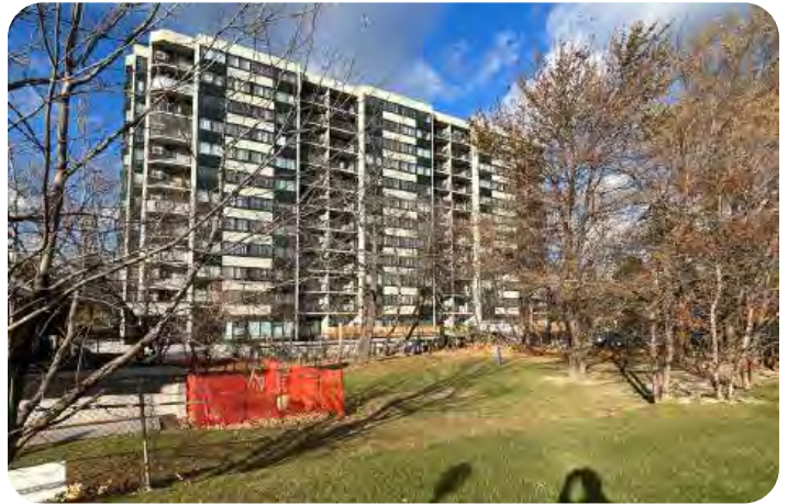
Rear of 1771 and 1773 Jane Street, looking north
